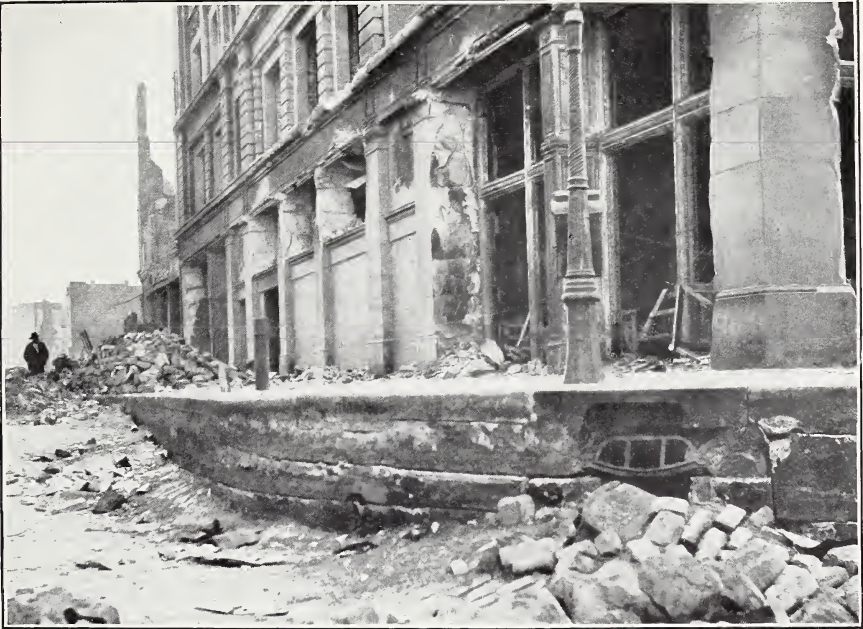
A. SUBSIDENCE OF STREET IN FRONT OF ÆTNA BUILDING. SAN FRANCISCO.
